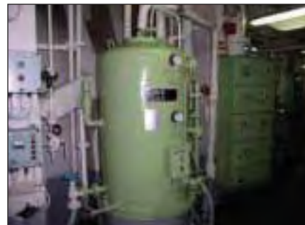
▲ Oily water separator
